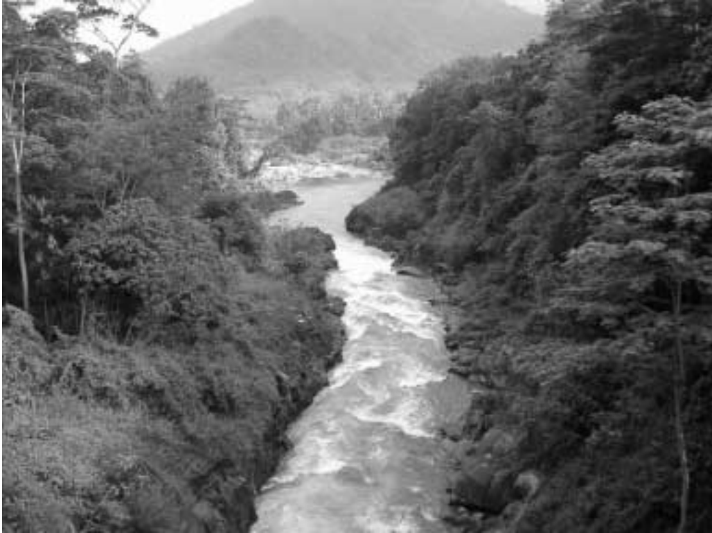
The Main Dam Site (looking downstream)
