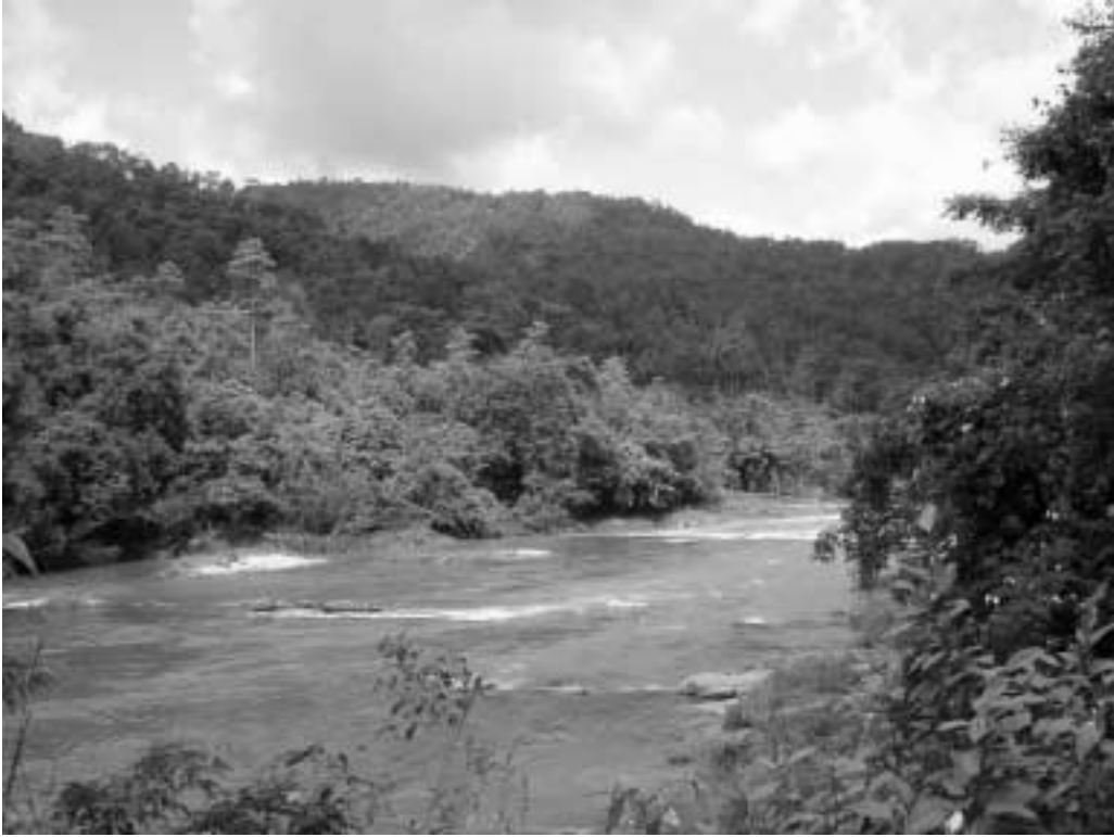
The Powerhouse Site (looking from the right bank)
