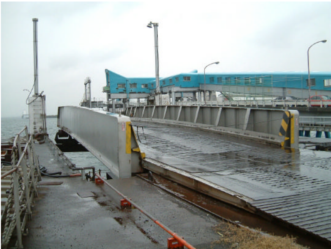
Figure A8.3.5 Movable Bridge (2)
