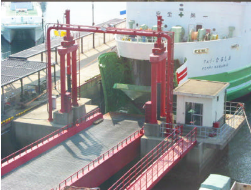
Figure A8.3.4 Movable Bridge (1)
