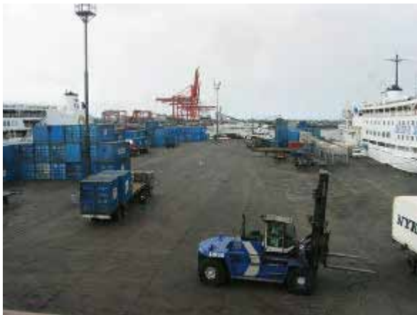
Manila North Harbor (Pier 4, PPA)
