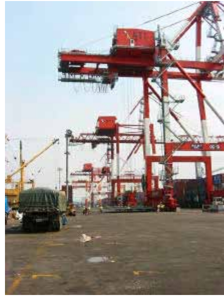
Manila South Harbor (Pier 5, PPA)
