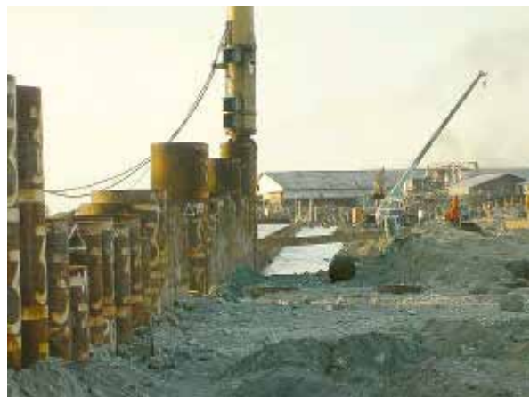
Mindanao Container Terminal (MCT, PIA) * under construction
