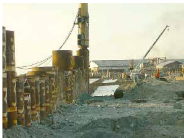
Mindanao Container Terminal (MCT, PIA) * under construction
