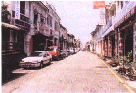
Road width of a collector (Lrg Hang Jebat) is about 9-12 m. which is barely wide enough for parking, traffic movement and pedestrian walkways.
