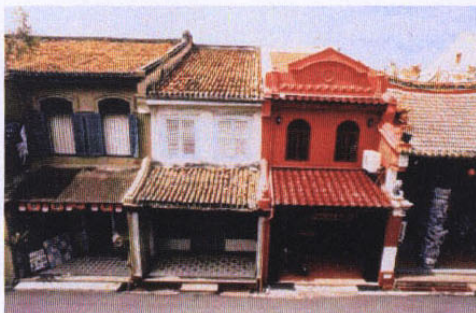
Building façade – Variety of Chinese and European Architectural Elements
