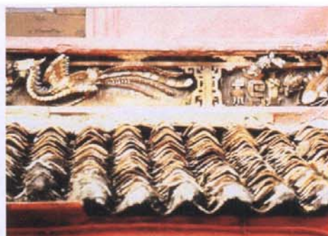
Building façade – Detail Freeze with colourful 'Chai Hui'
