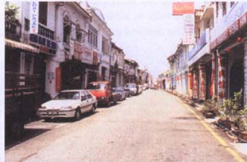
Road width of a collector (Lrg Hang Jebat) is about 9-12 m. which is barely wide enough for parking, traffic movement and pedestrian walkways.
