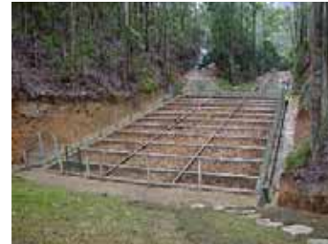
Leachate treatment facility
