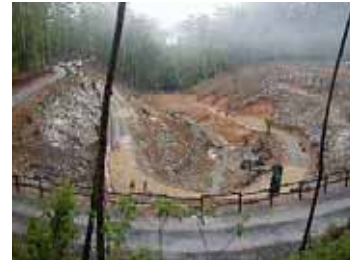
Relocation of existing waste & Cover soil
