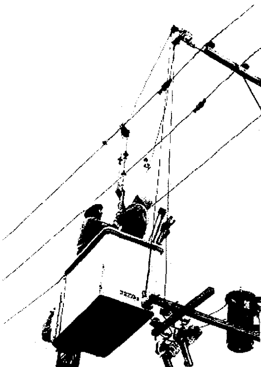
Fig. 2.3 - 5 Method of indirect hot-line work for joining high voltage mains and branch lines together halfway between poles
