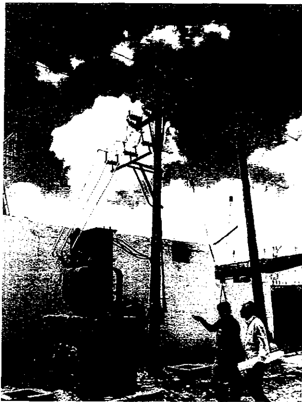
GIS Data Collection at Site
