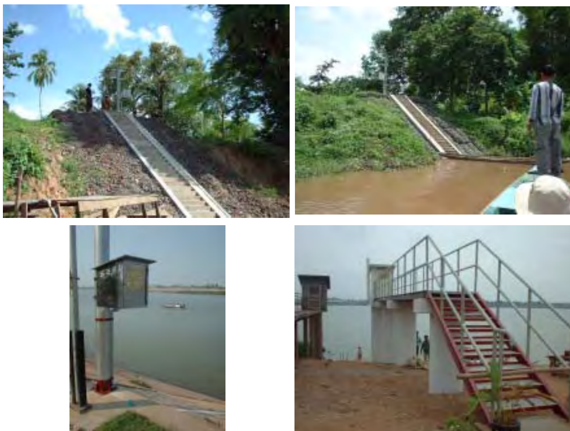
Fig. II-1-3 Locations of Four Stations in Cambodia and Overview of Improvement Works
