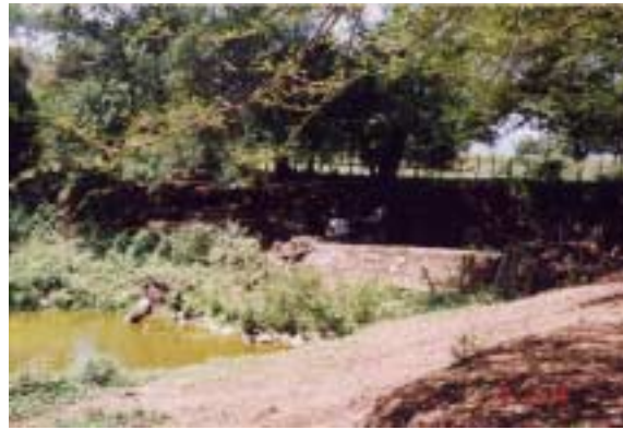
Concrete Weir at Entrance of Olomega Drainage (Rio Pelota)
