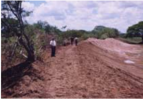
Existing Dike at Middle Reach of San Miguel River
