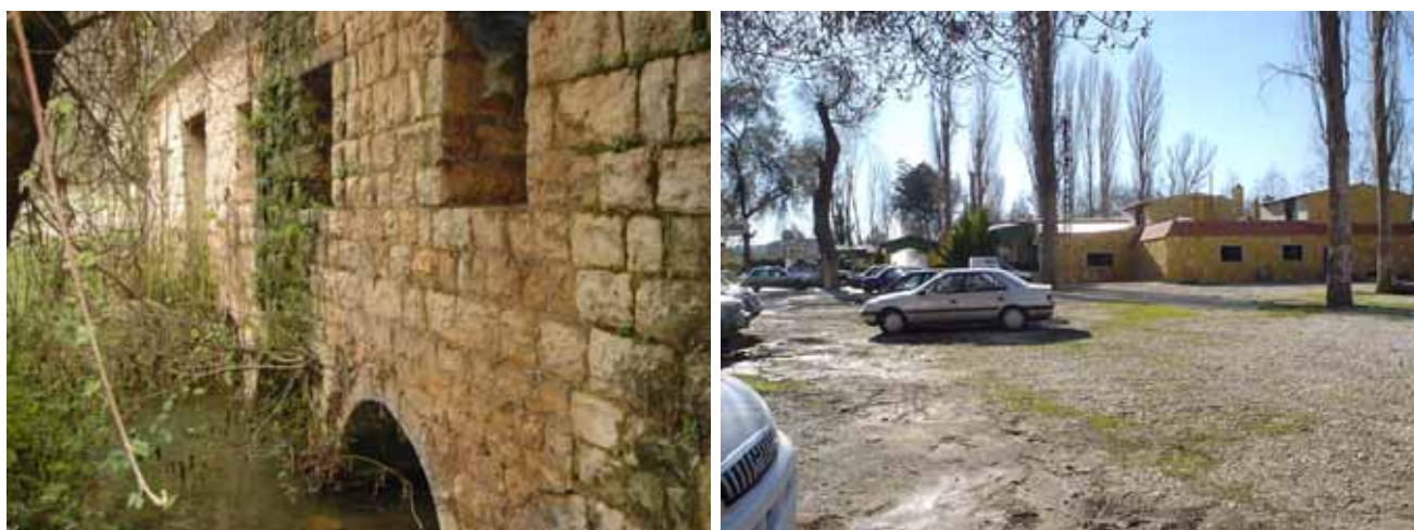
Photo 3.3.1 Abandoned Watermill Building and Proposed Site of Gold Souk
