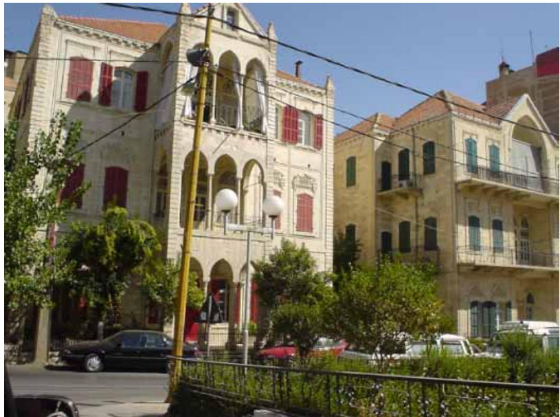
Photo 3.3.2 Zahle Heritage Buildings
