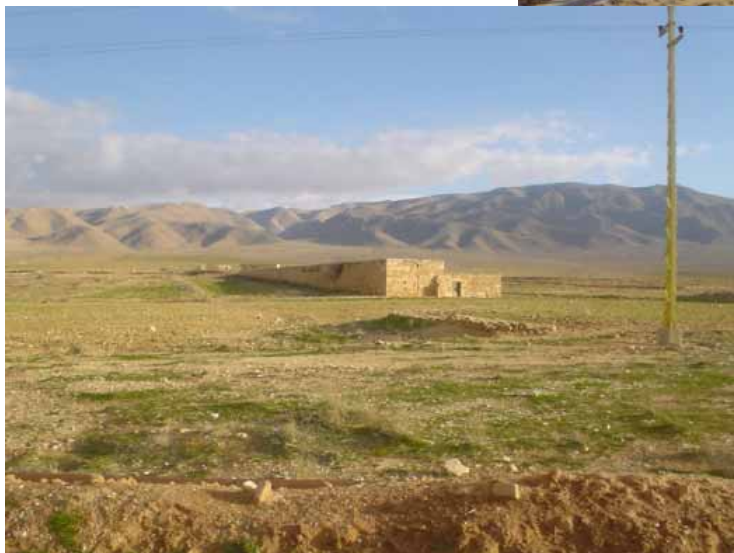
Photo S6 Watermill ruin in Qaa, North Bekaa
