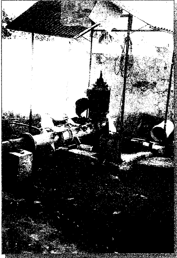
REGION 11 Davao Del Norte Municipality of Carmen Carmen Water District Production Well No. 1 Brgy. Tubod
