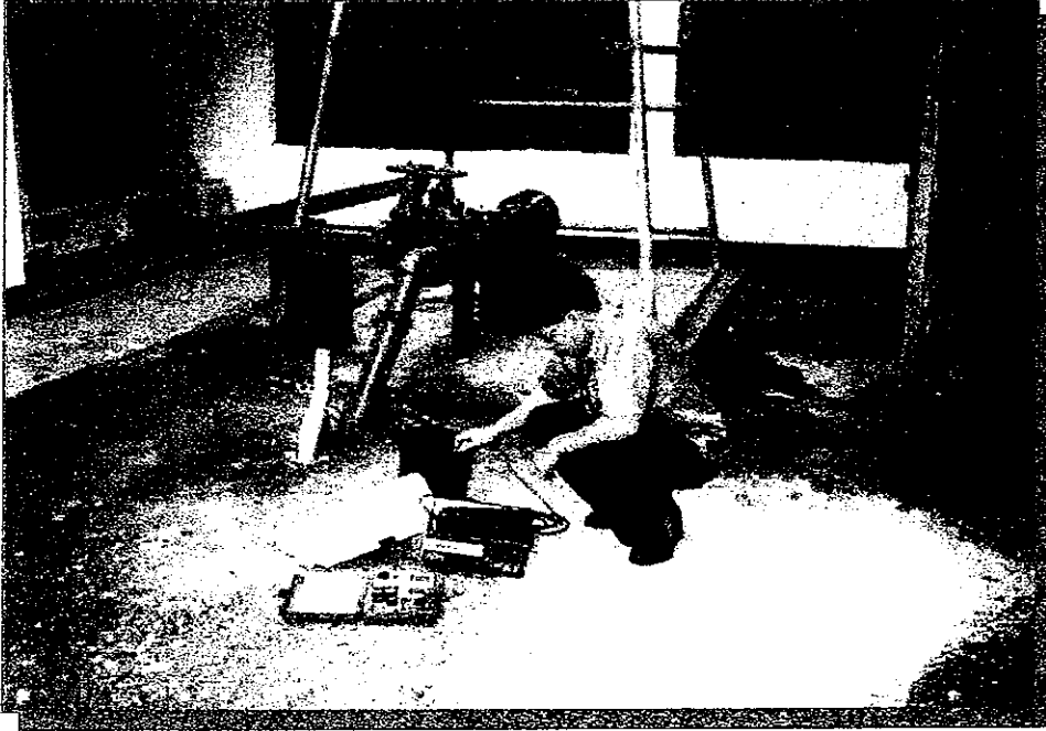
CARAGA Agusan Del Norte Municipality of Buenavista Buenavista Water District Production Well No. 1
