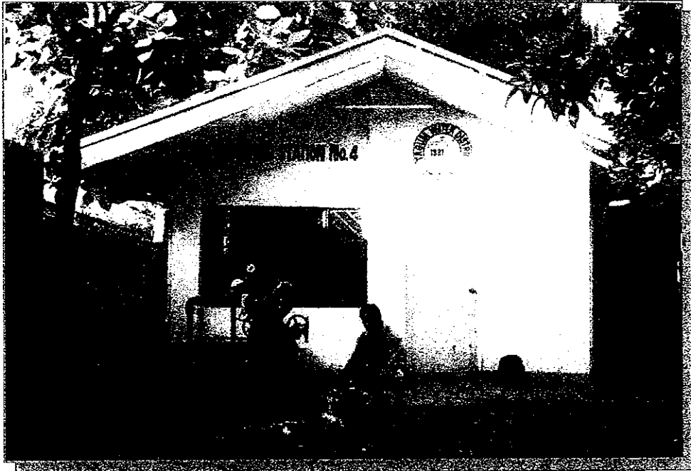
REGION 11 Davao Del Norte Municipality of Tagum Tagum Water District Well No. 4 Visayan Village
