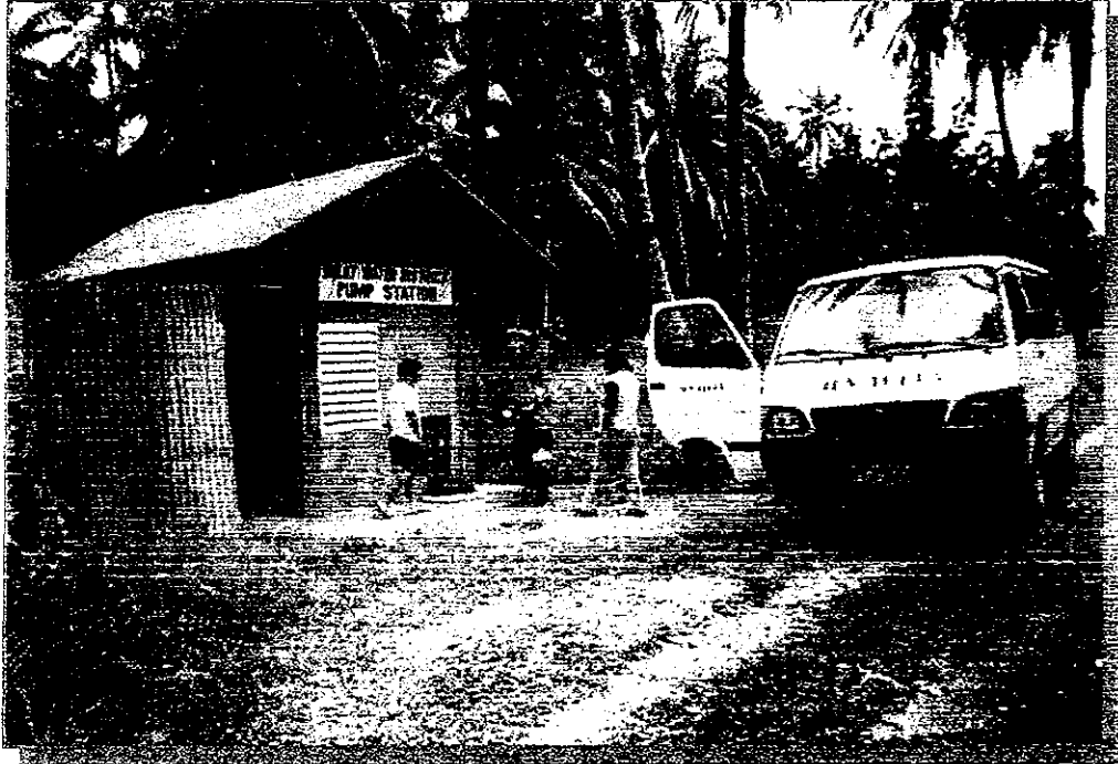
REGION 8 Eastern Samar Municipality of Sulat Sulat Water District Upper Sulat Well Brgy. Upper Sulat
