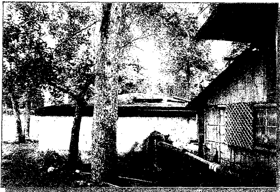
REGION 6 Iloilo Municipality of Barotac Viejo Barotac Viejo Water District BVWD Pumping Station Brgy. San Lucas
