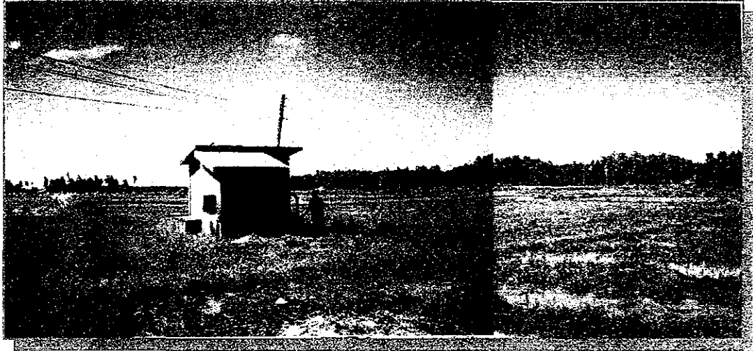
REGION 7 Bohol Municipality of Talibon Talibon Water District Pump Station No. 4 Brgy. San Jose
