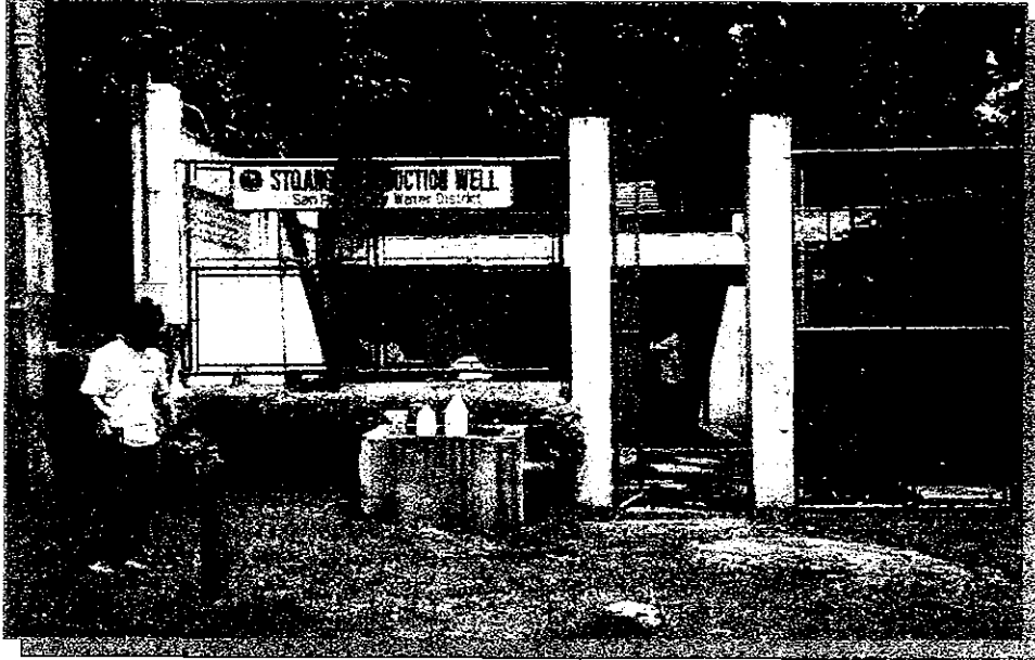
REGION 4 Laguna Municipality of San Pablo San Pablo City Water District Sto. Angel Production Well Brgy. Sto. Angel
