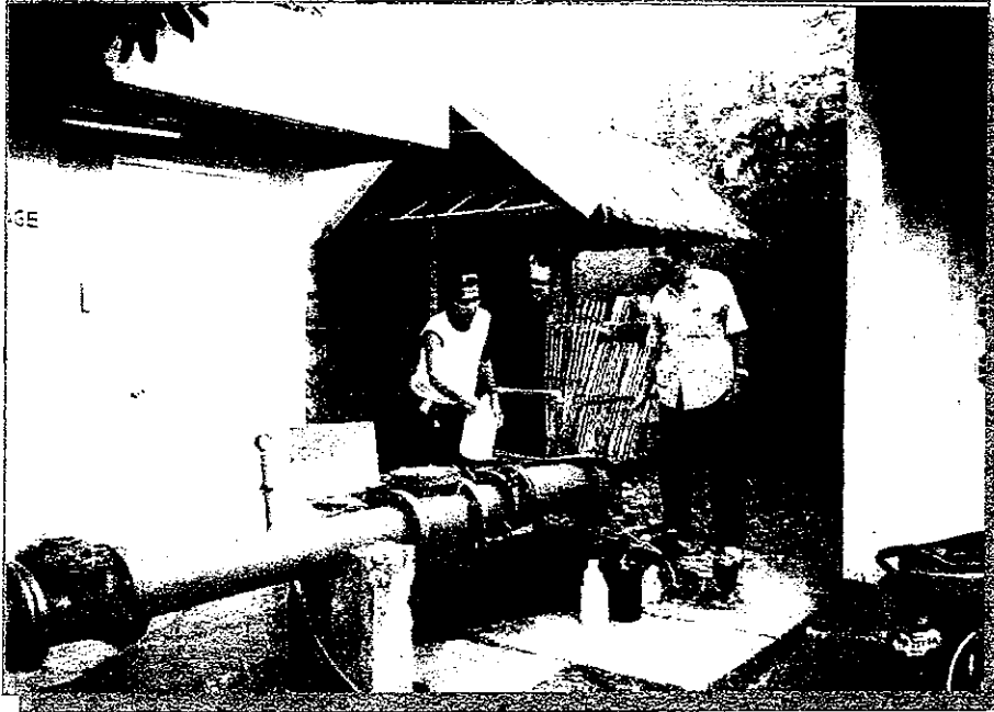
REGION 7 Negros Oriental Municipality of Dumaguete Dumaguete City Water District Deepwell No. 5 Brgy. Junob
