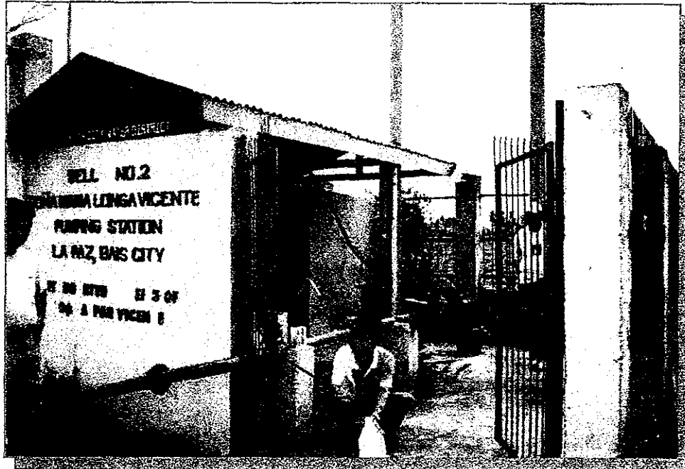
REGION 7 Negros Oriental Municipality of Bais Bais City Water District La Paz Well No. 2 Brgy. La Paz
