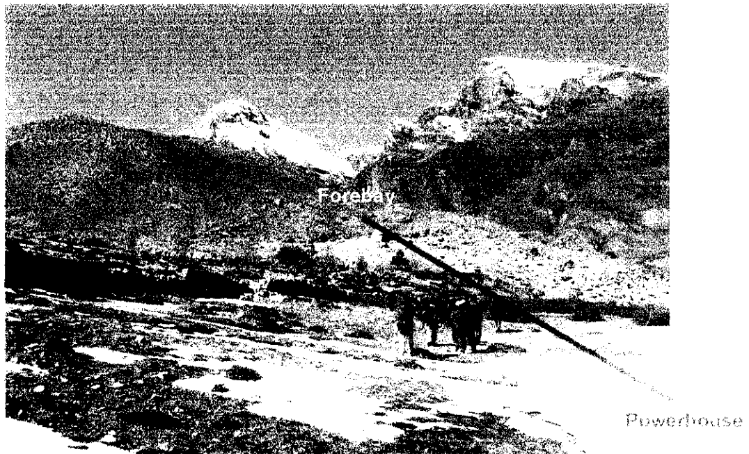
View of forebay, penstock alignment and powerhouse site
