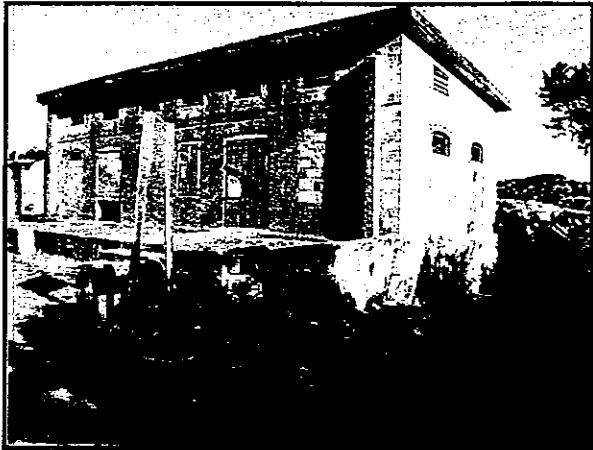
Photo-12 Historical building
