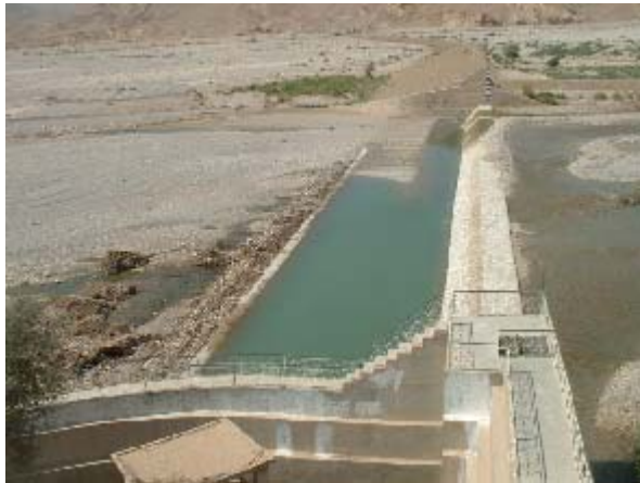
Bolon Weir Irrigation Scheme ㉔
