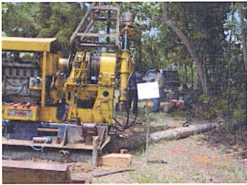
Start of Drilling, January 16 2004
