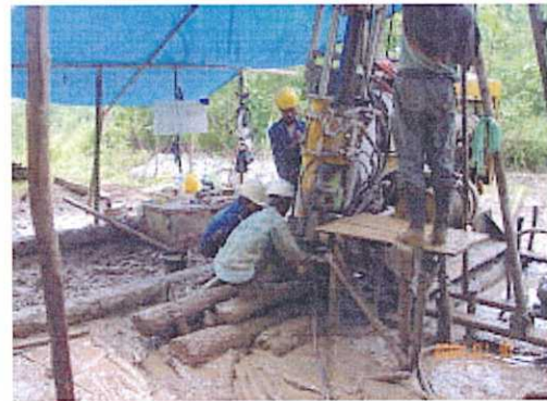
Pulling out NQ rods to change NQ bit
