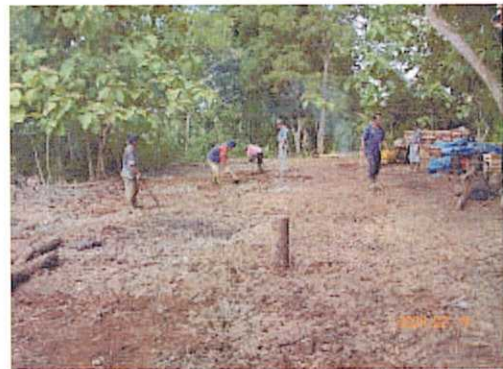
Reclamation after drilling
