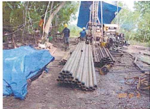
Pulling out NW Casings
