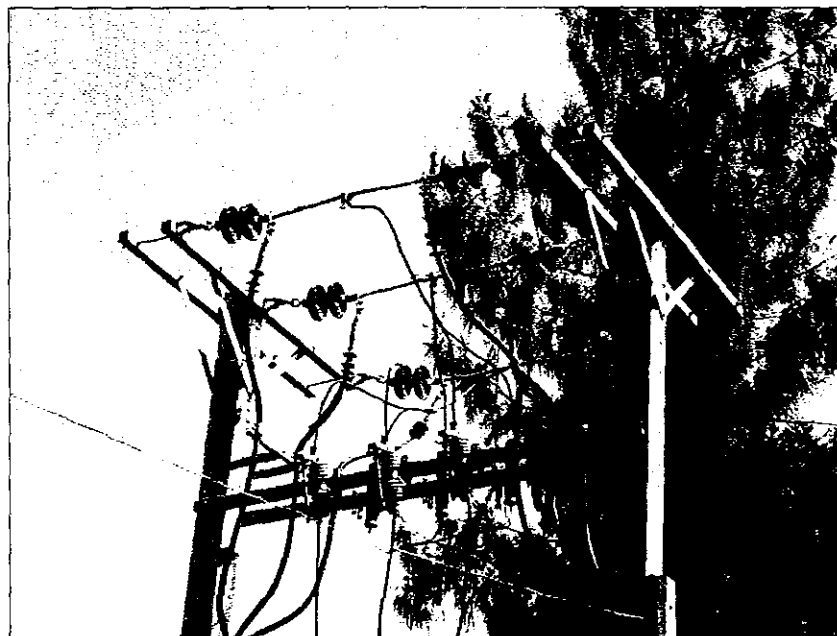
TRANSMISSION LINES IN PHNOM PENH AREAS
