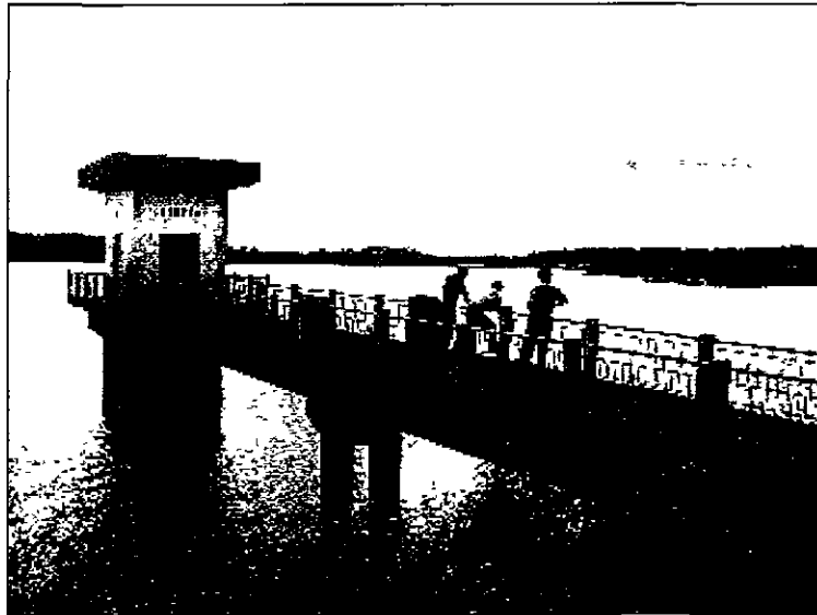
O Chum 1 intake tower
