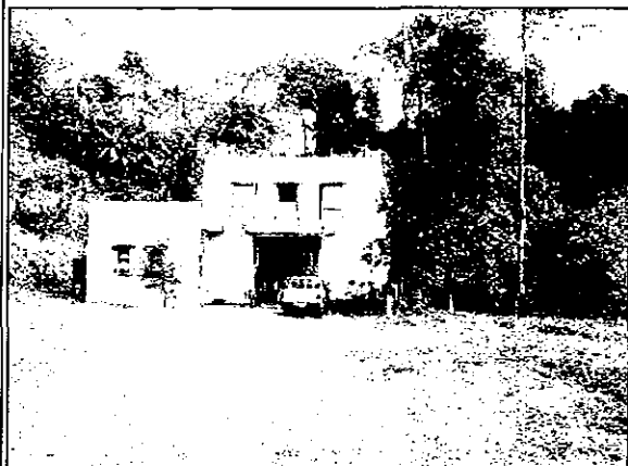
O Chum 2 powerhouse building
