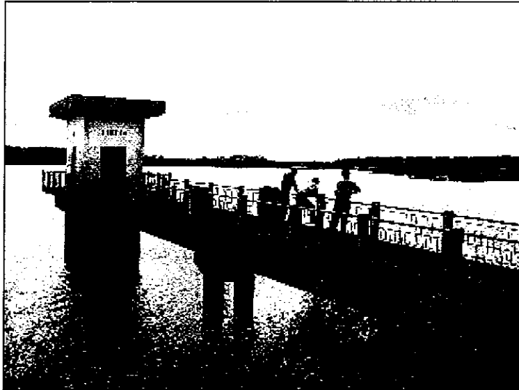
O Chum 1 intake tower
