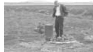
This well is an example of groundwater use in the Study Area. It is said that before it was artesian but recently constructed well head to use the water, due to the drought.
