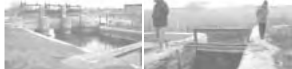
Diversion Weir ( from upstream side) Left Canal Intake (from downstream side) This weir locates in Ravansar City, just 1.0km down from the Ravansar Spring. "irrigation canals extend to both right and left sides for each I&D schemes."
