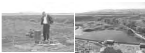
This well is an example of groundwater use in the Study Area. It is said that before it was artesian but recently constructed well head to use the water, due to the drought.
