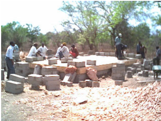
View of Construction (Multi-purpose Shed) (Mwanabwito)
