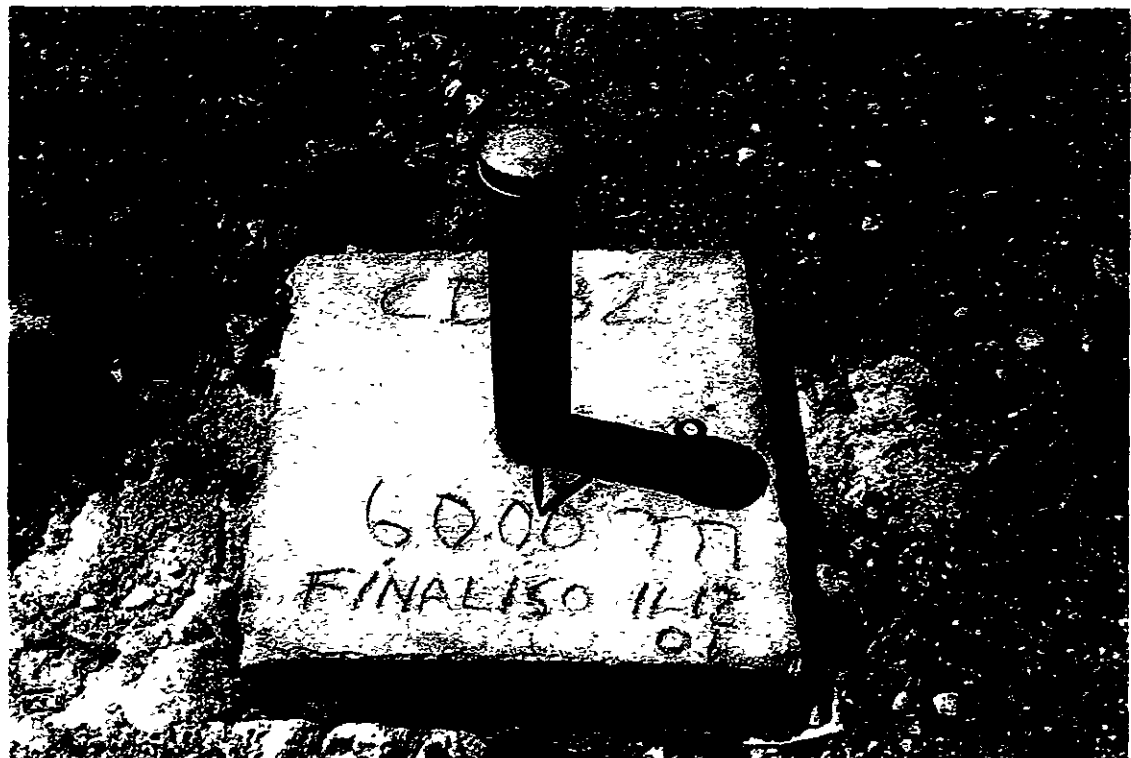
Photography No. 5 PIEZOMETER SURFACE PROTECTION
