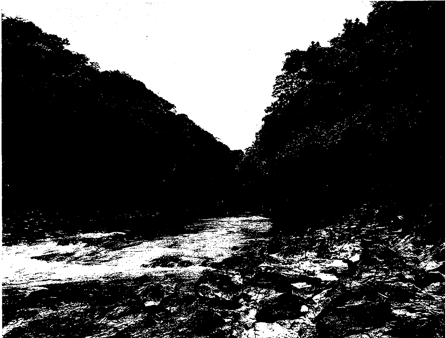
El Chaparral Dam Site (View from Downstream)
