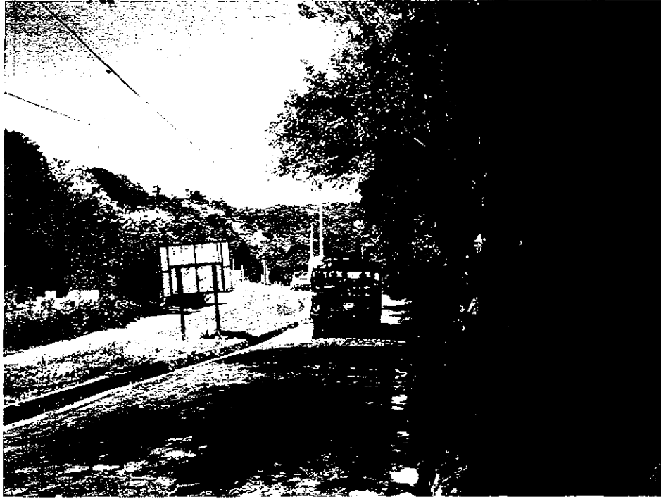
Road Condition (El Trinfo, Turning Point from Pan-American Highway)
