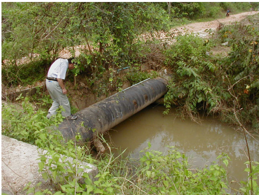
Photo A10-3 Location No.1
