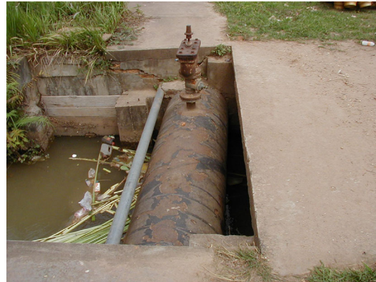
Photo A10-4 Location No.2
