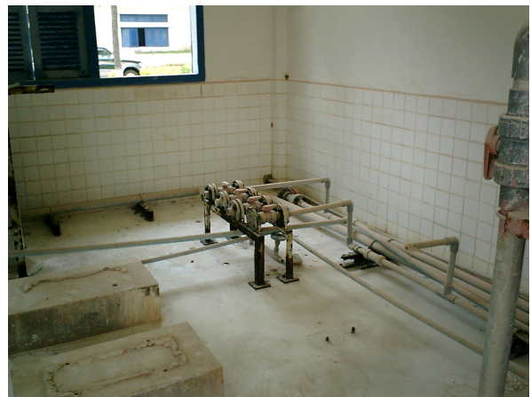
Malfunctioned Hypo Feeding Equipment
