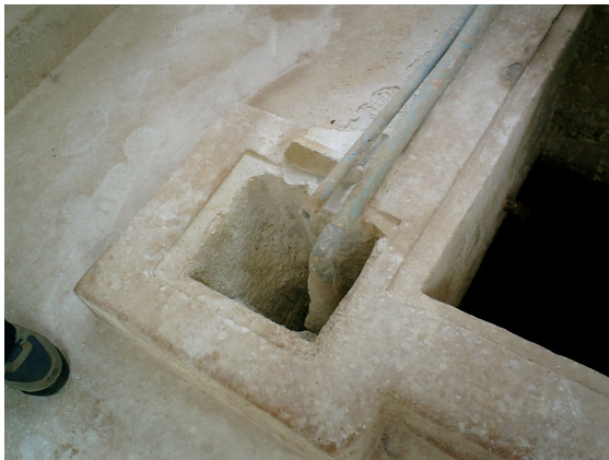
Hypo Dosing Point by Gravity Flow at the Clear Water Reservoir due to Malfunctioned Feeding Pumps
