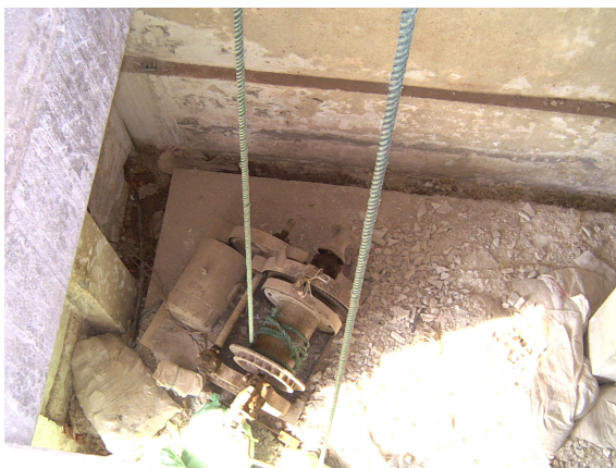
Malfunctioned Monorail System in Alum Storage Yard
