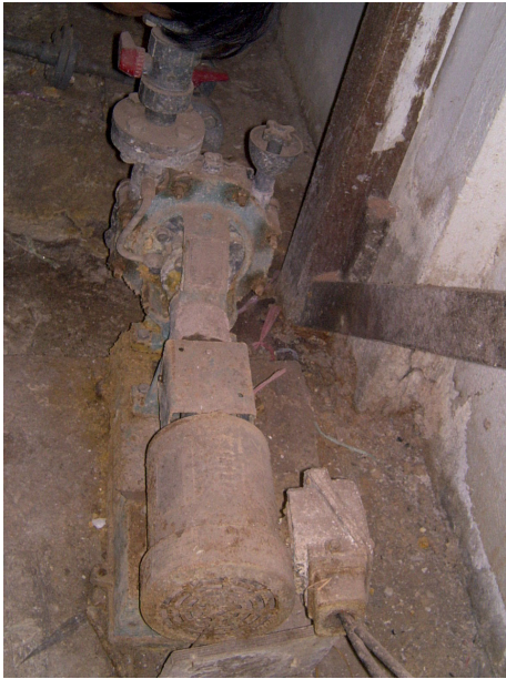
Malfunctioned Alum Circulation Pump
