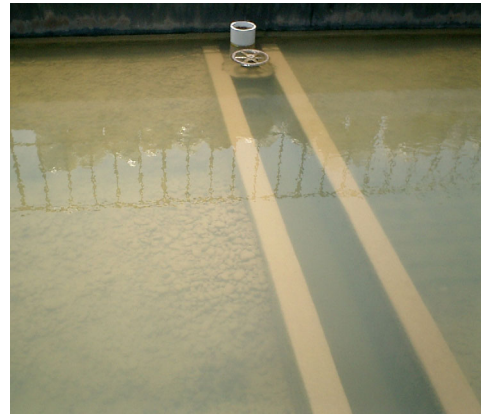
Gravel Filter (End of the Sedimentation Basin)
