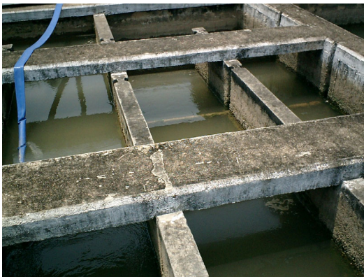
Flocculation Basin, Baffle Wall had been removed
