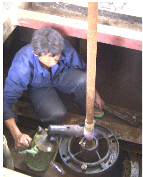
Shaft Extracting Work of Intake Pump
