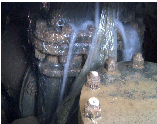
Malfunctioned Intake Discharge Valves Causing Heavy Leakage
