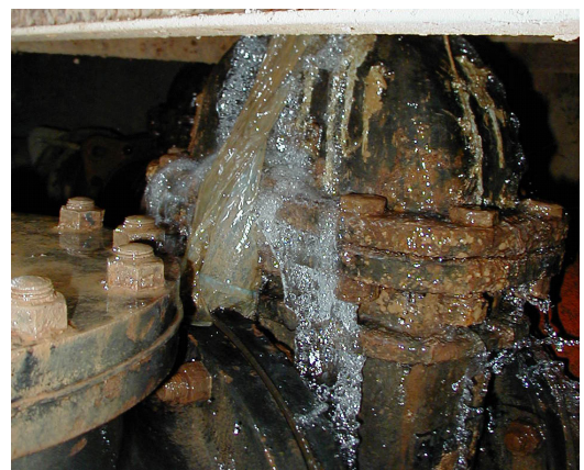
Malfunctioned Intake Discharge Valves Causing Heavy Leakage
