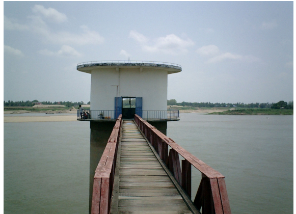
Intake Tower and Maintenance Bridge
