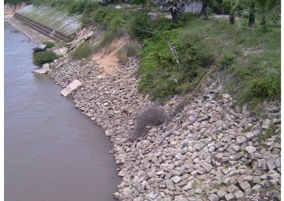
Upstream of Intake Tower, the Mekong River
