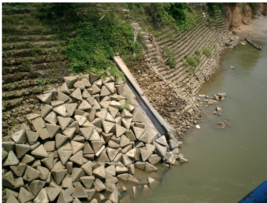
Down Stream of Intake Tower
