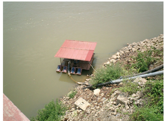
Intake Pump on Pontoon
