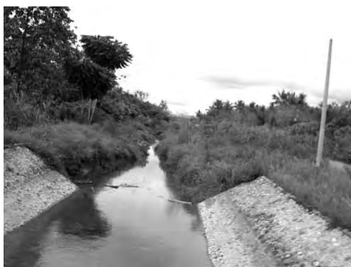
5. Canal Condition at 9.7 km point (BK Ki 10)
