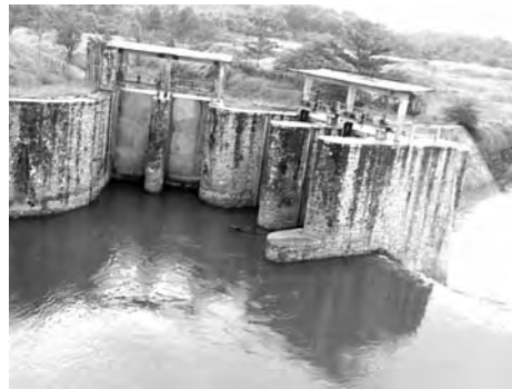
2. Headworks, Scouring Sluice (right) and Intake (left)
