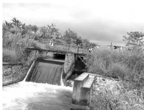
4. Off-take of Division Structure at 2.4 km point
