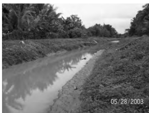
Condition of Earth Canal Section
