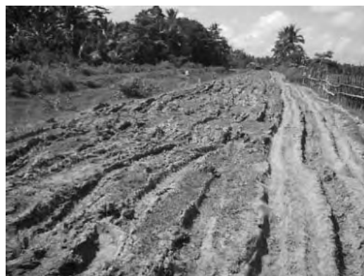
Condition of Inspection Road
