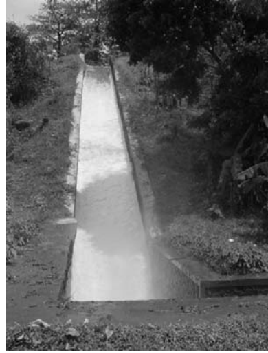
4. Chute Structure on Main Canal
