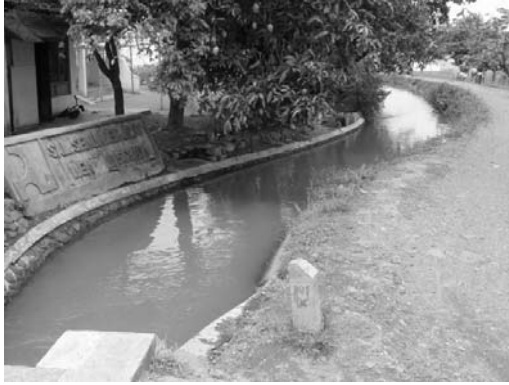
3. Beginning Point of Main Canal (HM 0+00)
