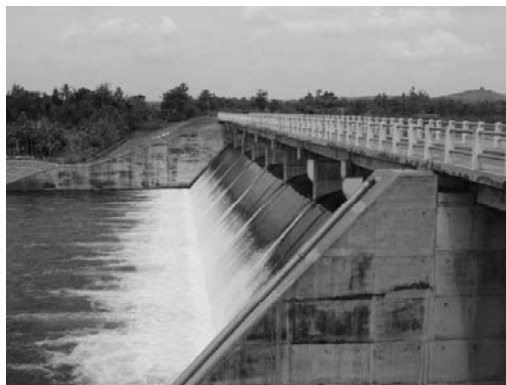
In Good Condition
