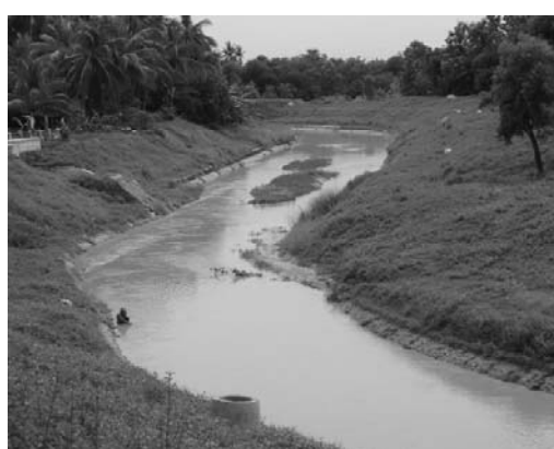
In Good Condition
