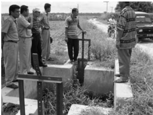
5. Condition of Terminal Facility (Out of Services)
