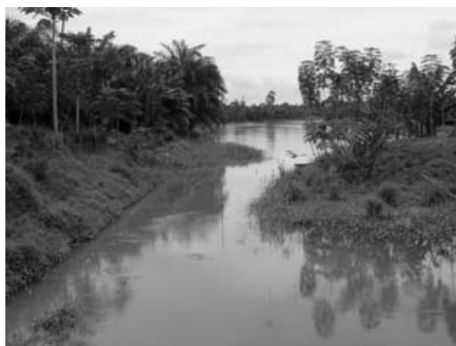
2. Inlet Channel of Intake from Asahan River (No removal of sediment and eroded earth)
