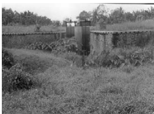
Sediments in front of Intake
