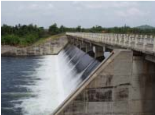
SIDOREJO Headworks (Central Java Province)
