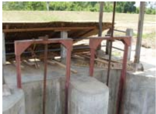
BANDAR SIDORAS Headworks (North Sumatra Province)
