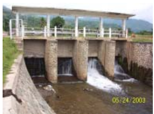
LAMASI KANAN Headworks (South Sulawesi Province)
