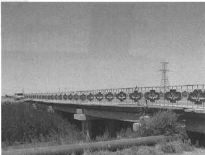
Km302 Bridge 5 x 9m section.
