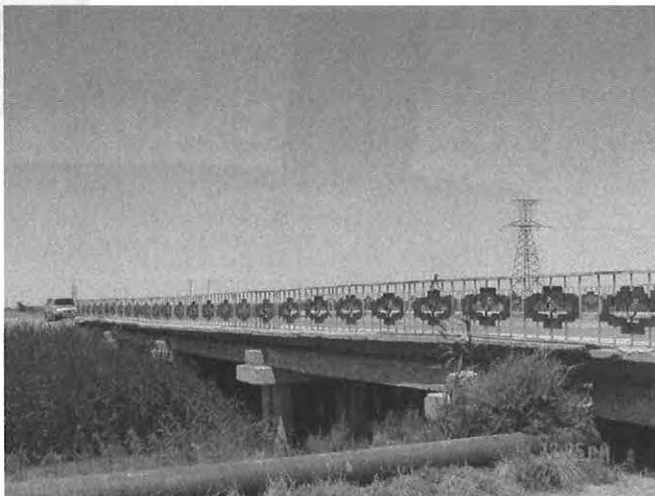
Km302 Bridge 5 x 9m section.
