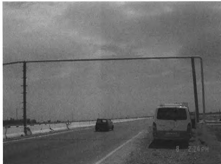
Km 188 150mm gas line 6.1m clearance.
