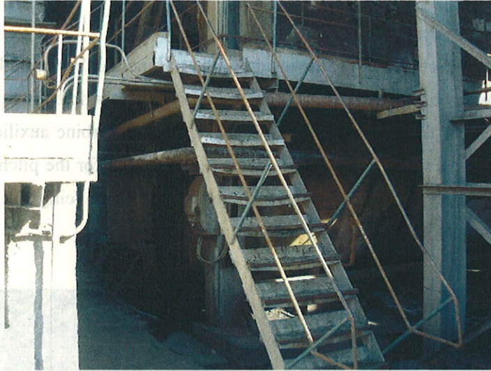
Picture 5.1-12 Stairs and Walkway Handrails
