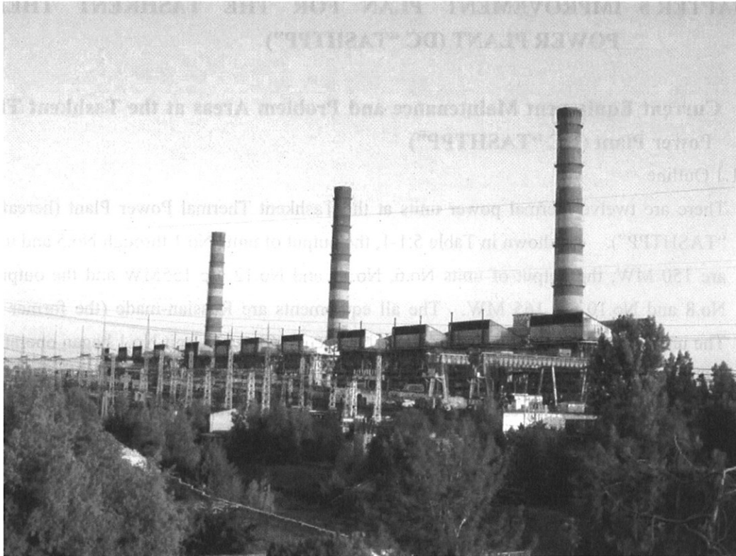
Picture 5.1-1 Existing Tashkent Thermal Power Plant
