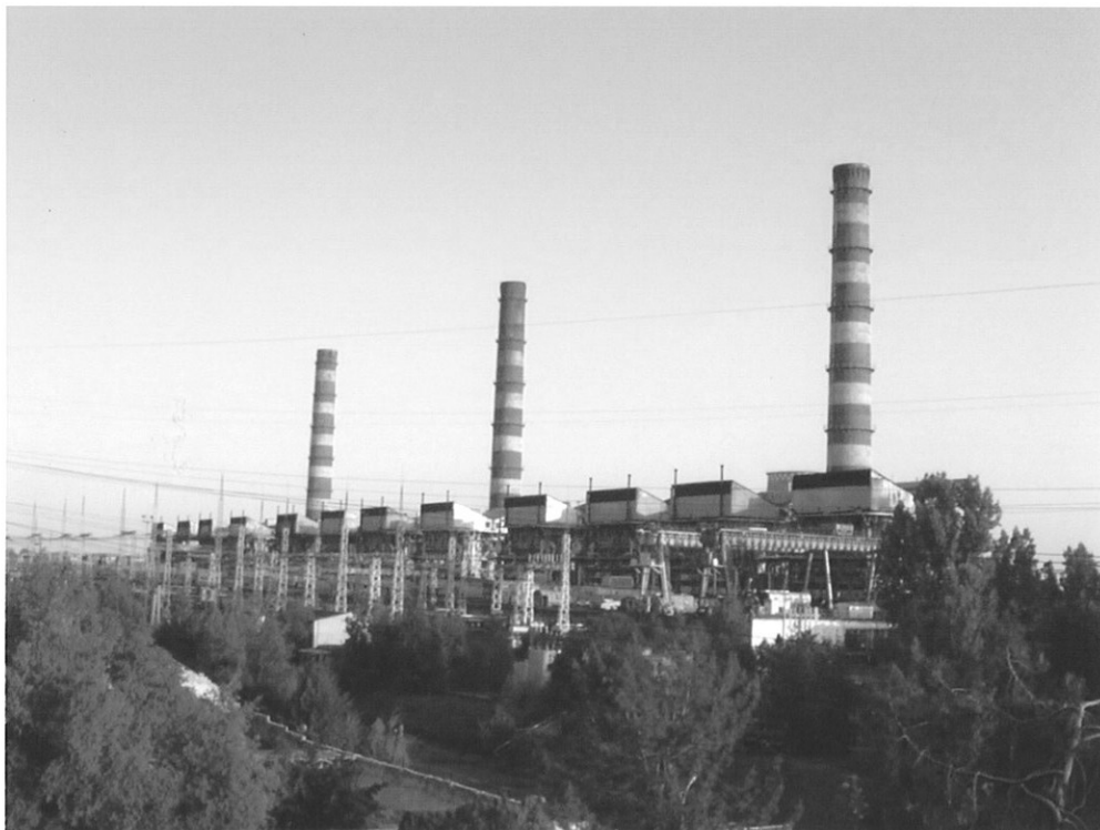
Bird's-eye View of Tashkent Thermal Power Plant (from Administration Building)
