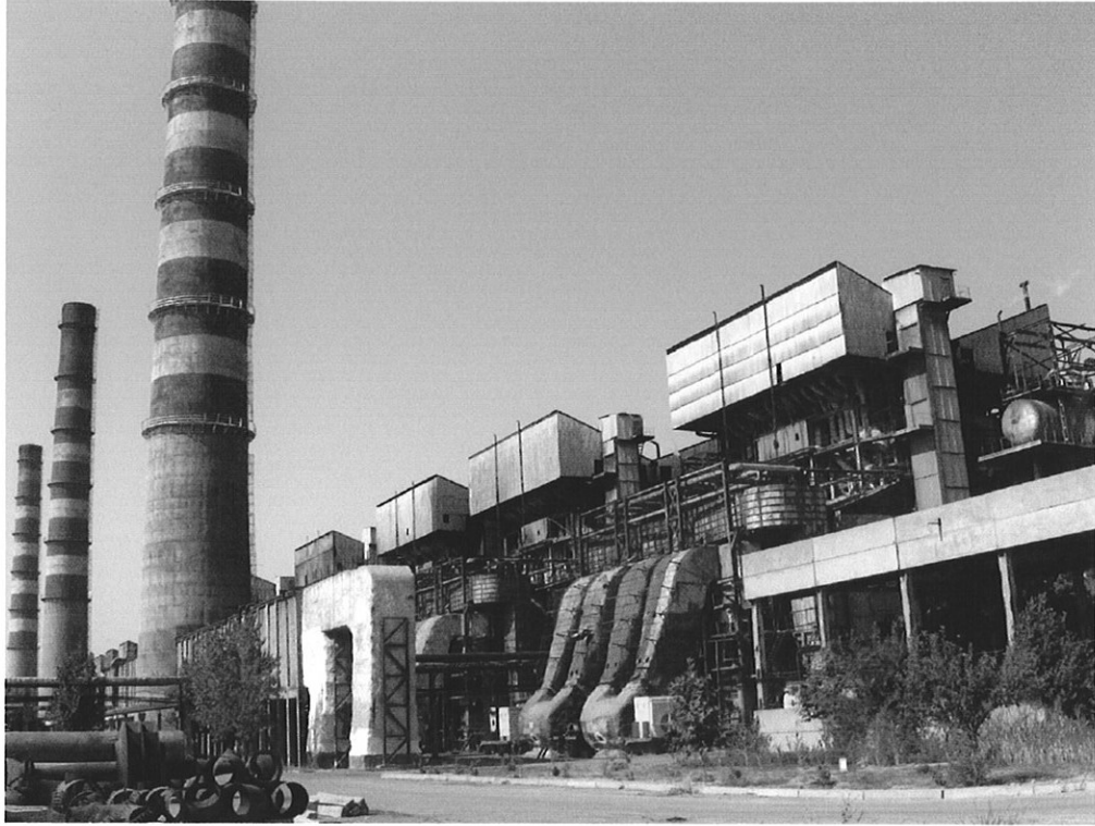
The Existing Boiler Equipments(Units 11 and 12 from right side)
