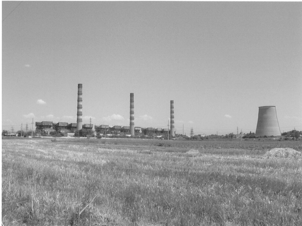
Bird's-eye View of Tashkent Thermal Power Plant
