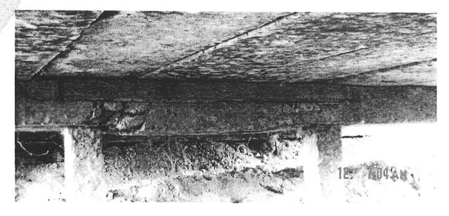
**Km 12.3** Bridge 4 x 6m section. Bridge requires repair to piers due to cracking.
