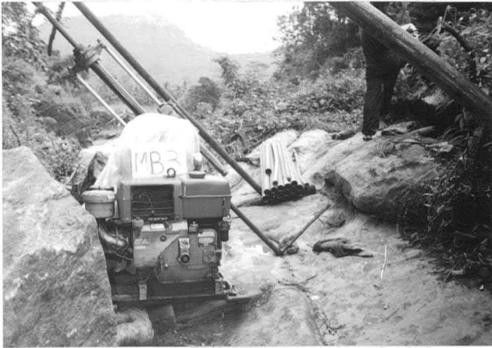
| Plate # 10: Drilling Location of MB-3 Total depth of hole: 50.00m
