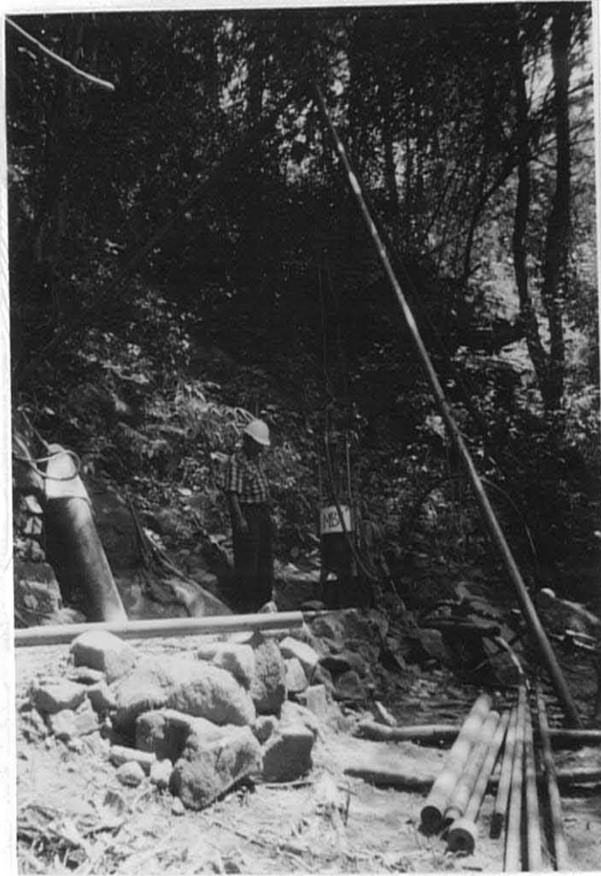
Plate # 4: Drilling Location of MB-1 Total depth of hole: 40.77m
