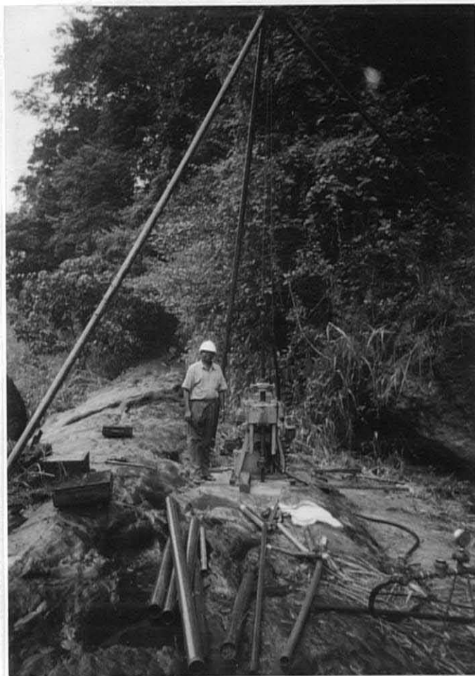
Plate # 7: Drilling Location of MB-2 Total depth of hole: 40.13m
