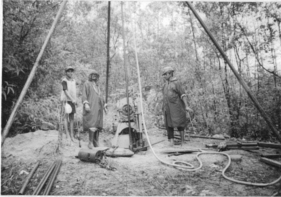
Plate # 25: Drilling Location of MT-2 Total depth of hole: 35.00m
