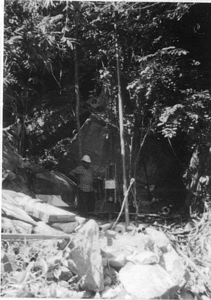
Plate # 13: Drilling Location of MB-4 Total depth of hole; 40.00m
