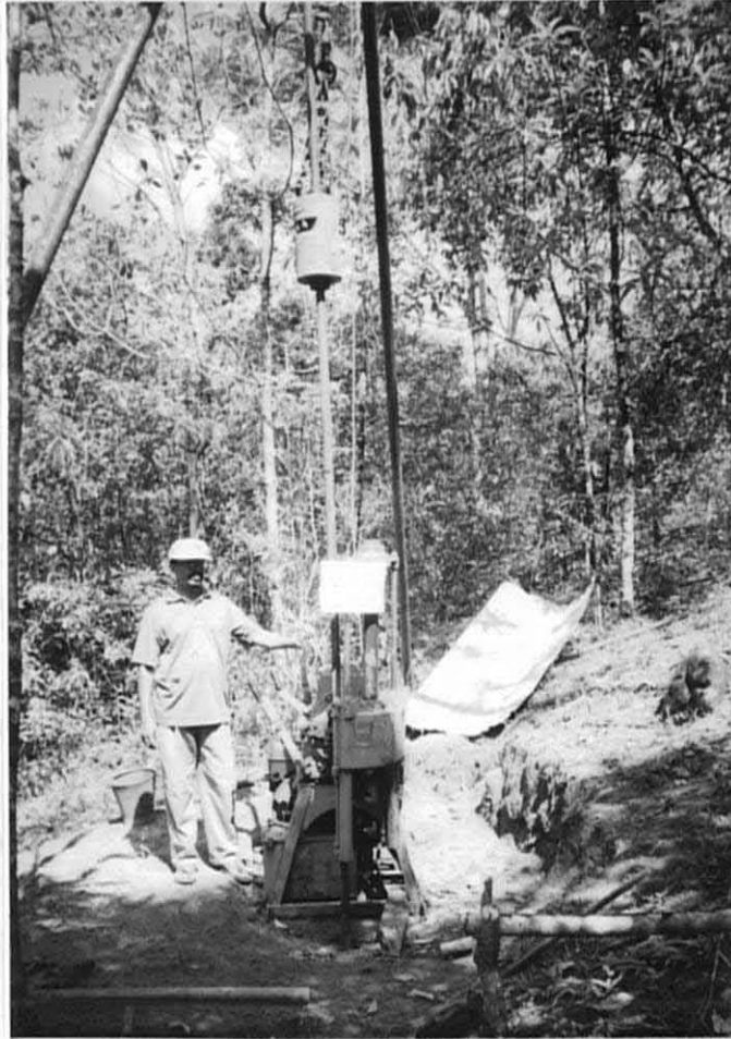
Plate # 27: Drilling Location of MT-3 Total depth of hole: 25.57m
