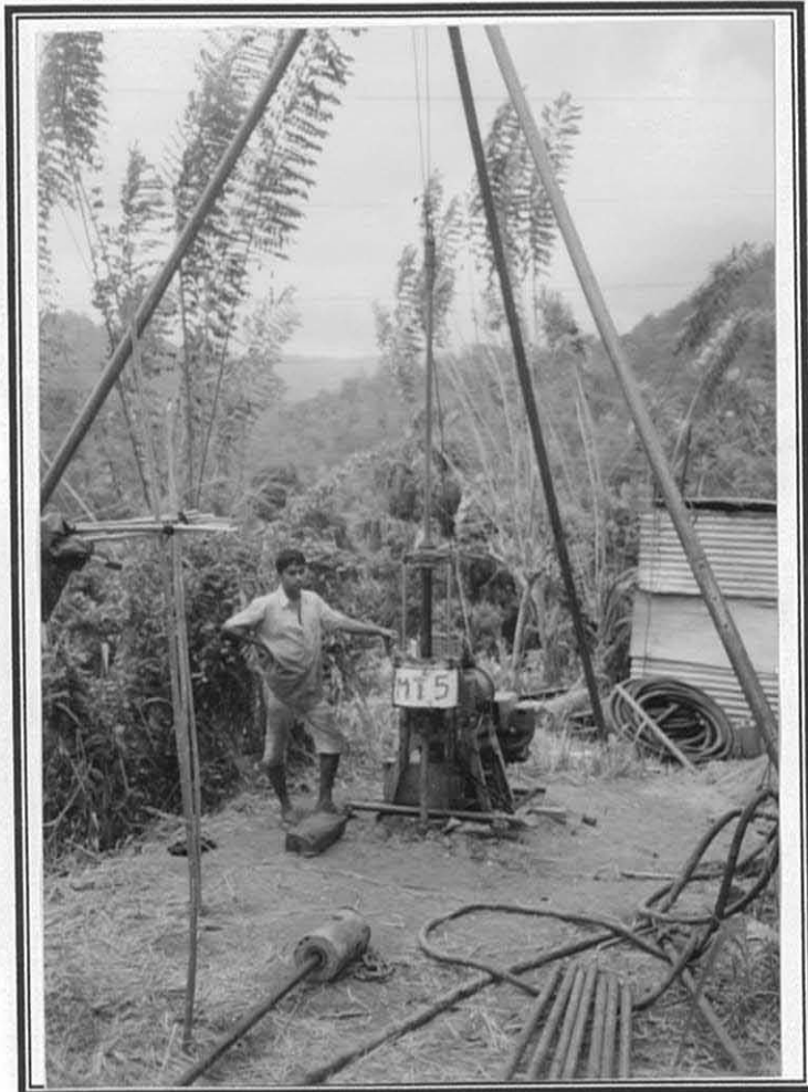
Plate # 12: Drilling Location of MT 5 total depth of hole 30.25m
