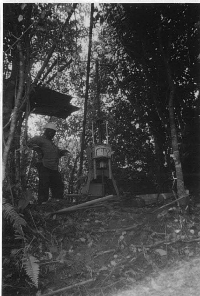
Plate # 19: Drilling Location of CT2 Total depth of hole: 15.50m
