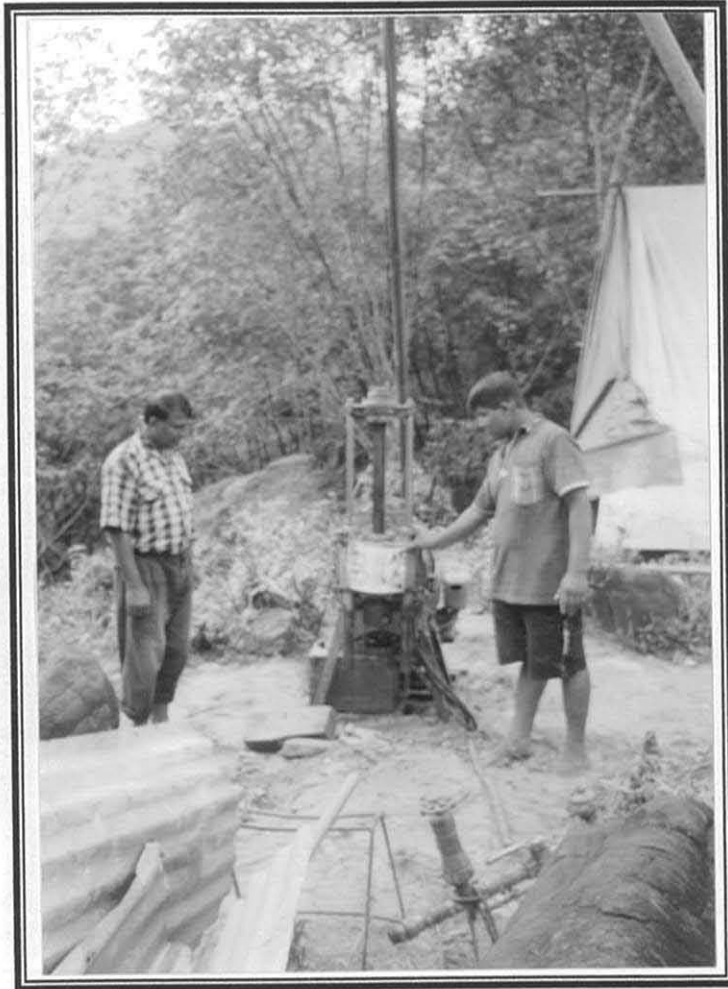
Plate # 28: Drilling Location of BQ 2' total depth of hole 25.10m
