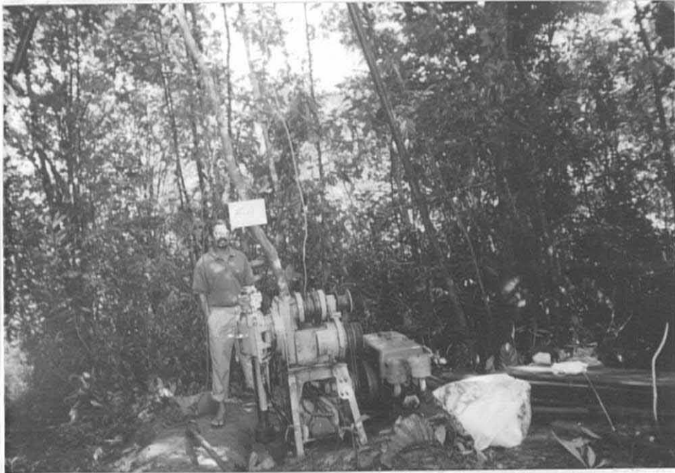
Plate # 30: Drilling Location of MT-4 Total depth of hole:30.55m
