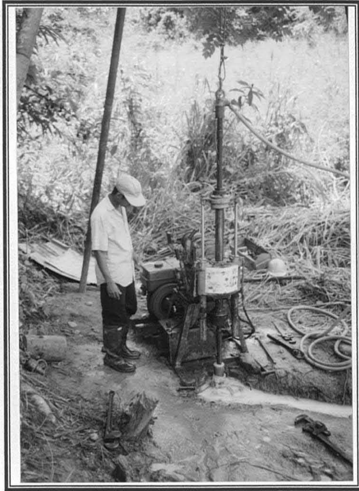
Plate # 9: Drilling Location of CT 4 total depth of hole 20.00m
