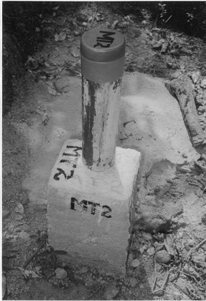
Plate # 25: Hole monument of MT-2 with cap
