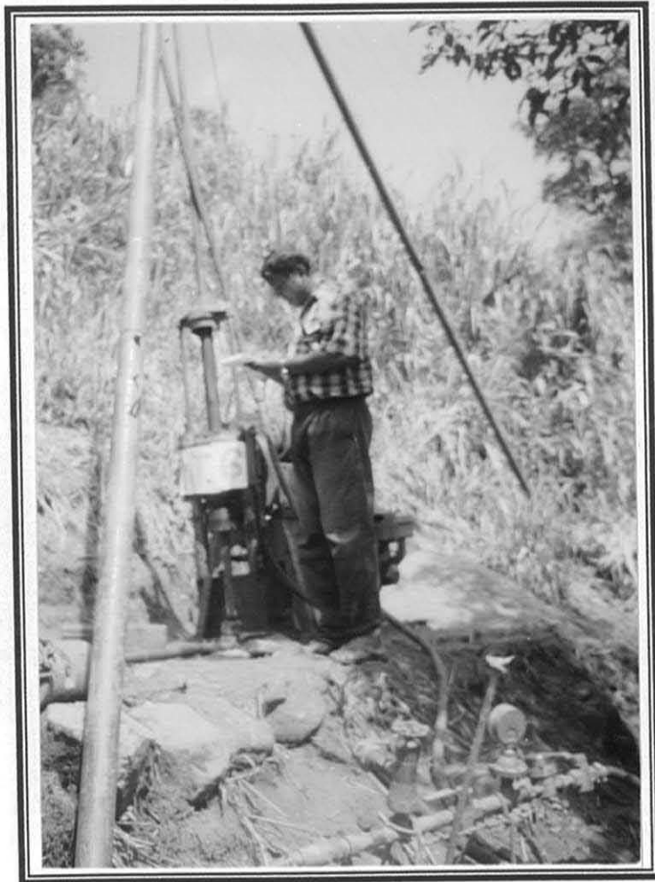
Plate # 15: Drilling Location of MT 6 total depth of hole 40.10m
