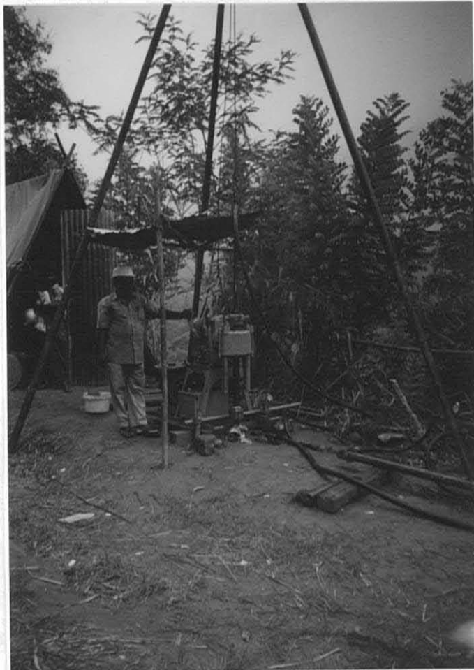
Plate # 22: Drilling Location of MT-1 Total depth of hole: 35.54m
