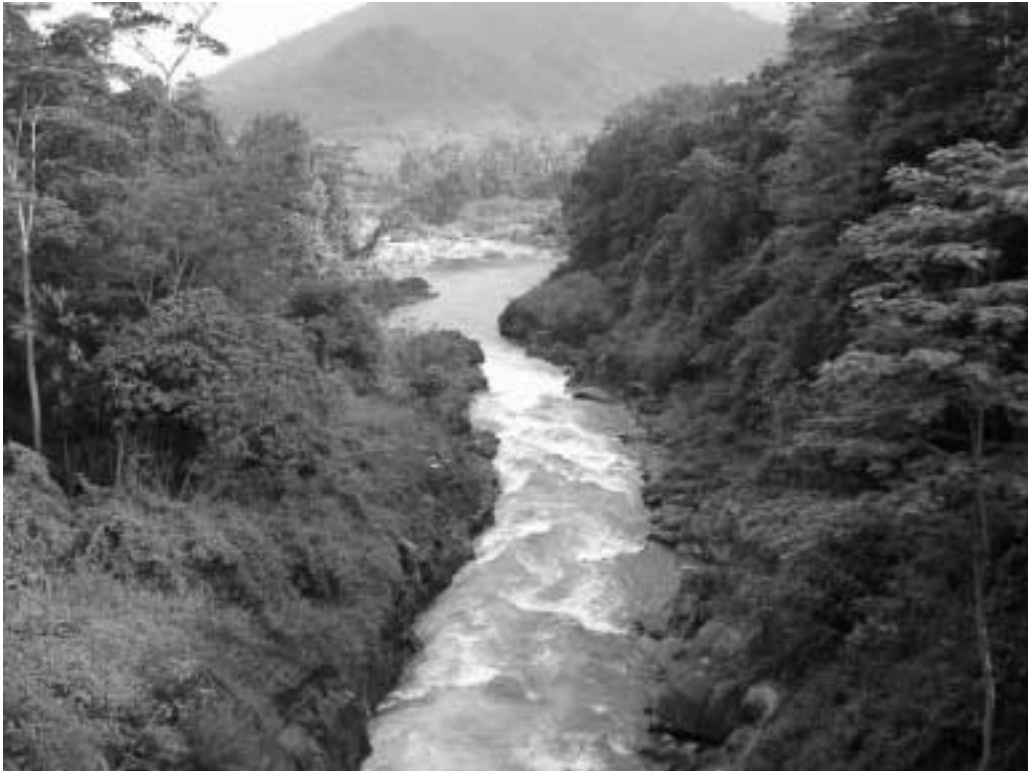
The Main Dam Site (looking downstream)
